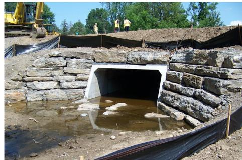
The client and the design team liked the rustic look of the existing culvert but after the determination was made that rehabilitation was not an option, thinking outside of the box ensued. What if we could preserve the look and feel of the stone culvert? The recycle/reuse concept came to be and the construction team was asked to dismantle the culvert. When the deconstruction process began, it appeared that this novel idea might not be practical.
